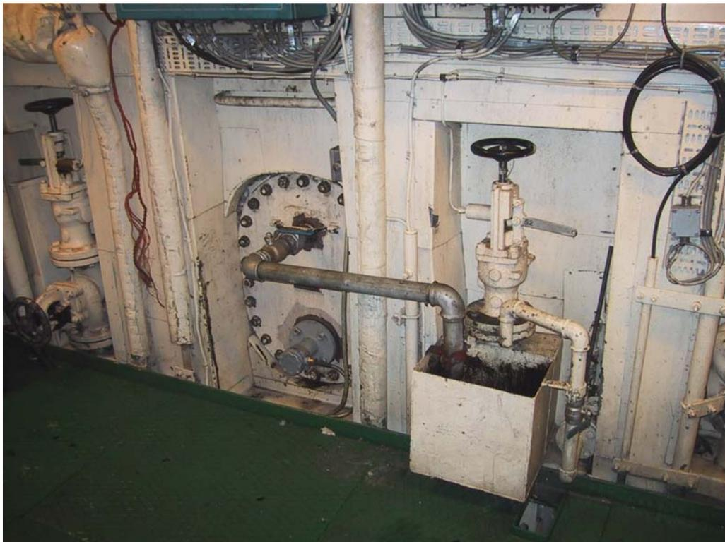
Fig. 11: Penetration through a manhole covers to a high tank.
